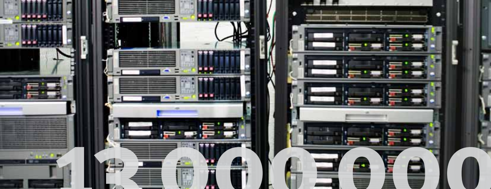
Server stack at ECDC
